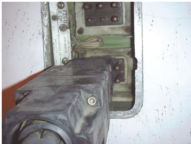
Example of incorrect connection (Boeing source)
