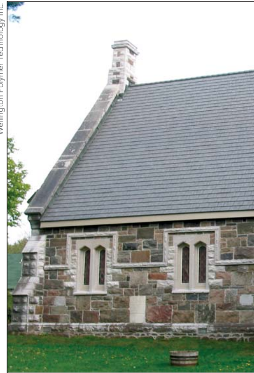
St. George's Church, a heritage site in Sutton, ON, sports an environmentally friendly Envirosake roof. The bioproduct has the same look as the old cedar roof it replaced.
